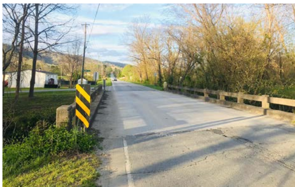
Image 14. Stream Crossing and Bridge on Jackson Rd (SR 1539)
