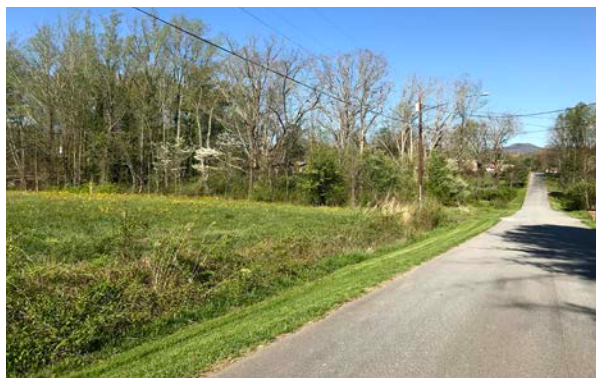
Image 15. Drainage Ditch Along Poteat St
